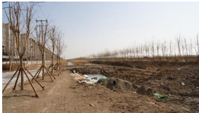
2. Houses face the park & ditch barrier
