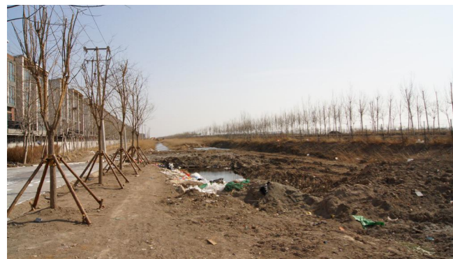
2. Houses face the park & ditch barrier
