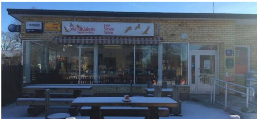
Figure 2 The building with café, postal counter, tourist information center and a local organization- Svartådalens Bygdeutveckling. By Kit Wa Lai, 2016.
