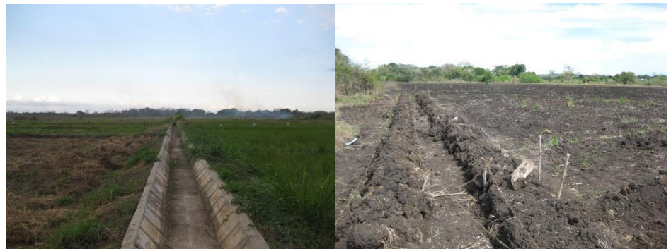
Figure 9. Left: Concrete irrigation canal in the rice scheme in Misasi. Right: Soil irrigation channel in the rice scheme in Kakora. (Photo: Agnar Kjeller).
