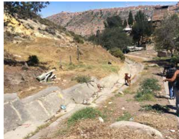
Canal in the west
