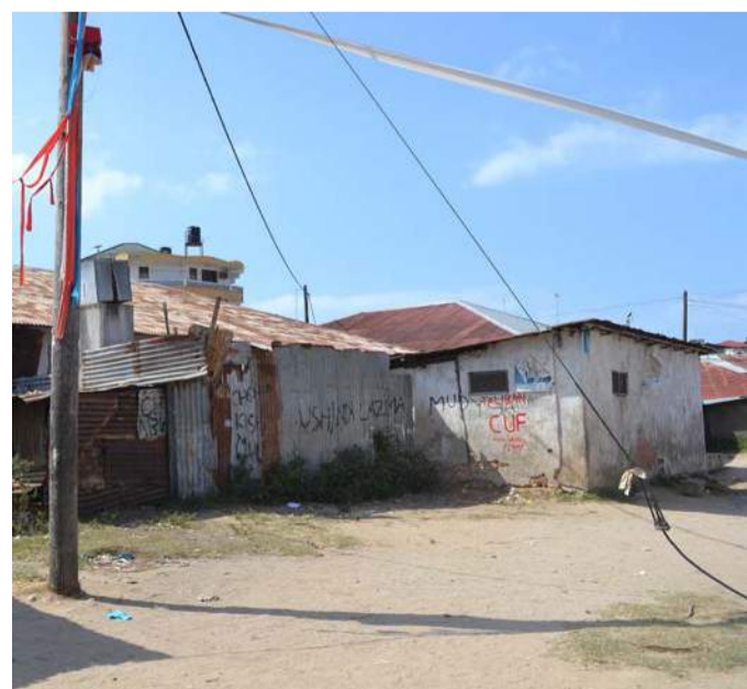
Electricity pole with a connected wire
