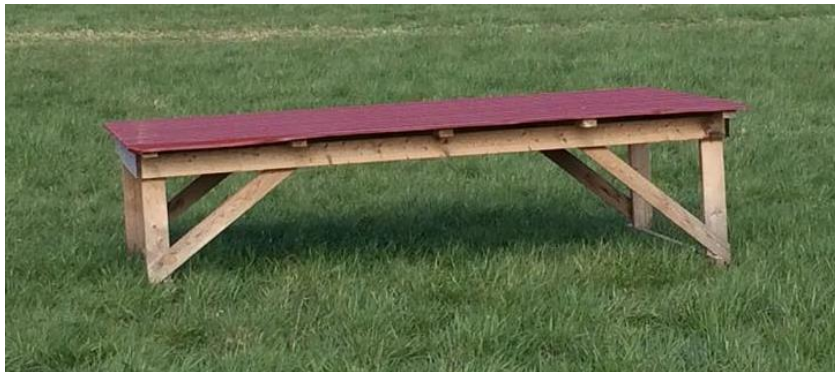
Figure 1. A shelter with a tin roof and four wooden legs
