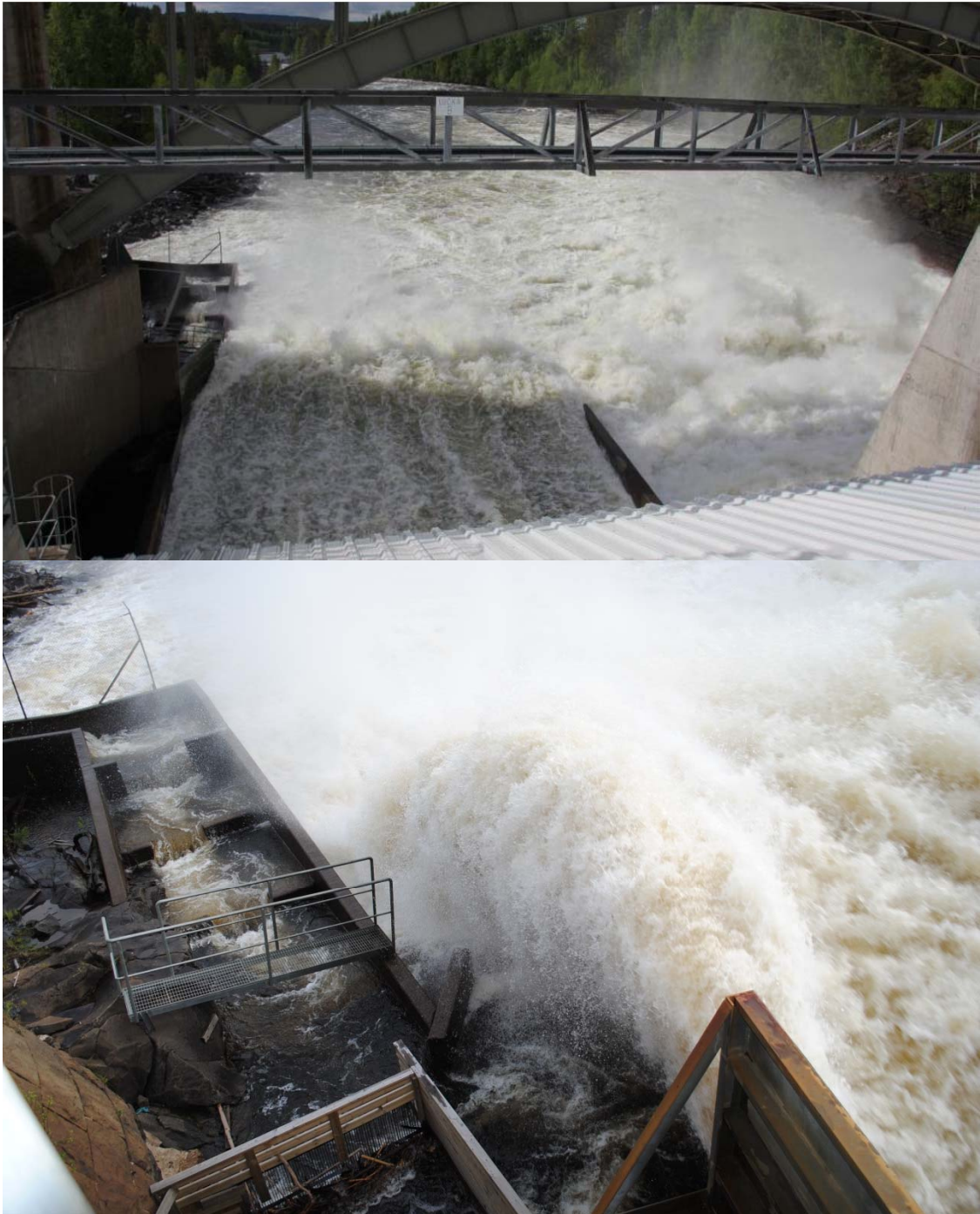
Figure 7. Picture showing the area below spill gate B where the water released from the spill gates hit the opening of the fish ladder (Photo: Linda Vikström).
