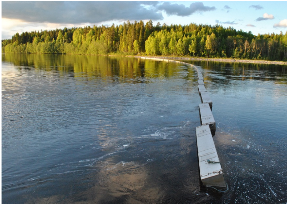
Figure 4. Picture showing the guidance structure that stretches from the north shoreline to the mid-section of the dam, thus guiding fish away from the power station (Photo: Linda Vikström).
