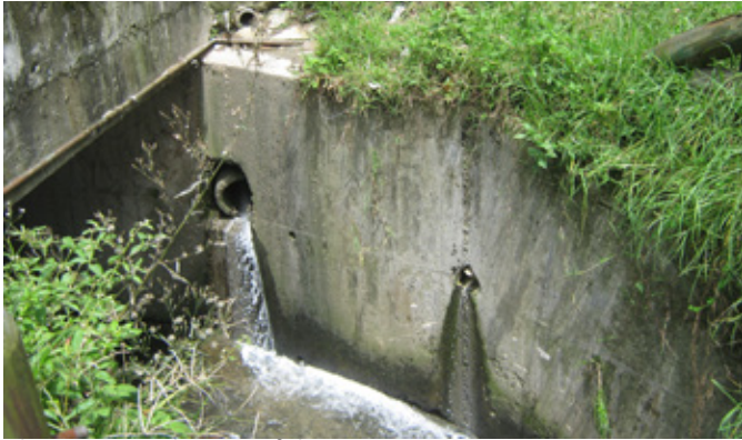
Photo 48. Canalisation of the rivers.
