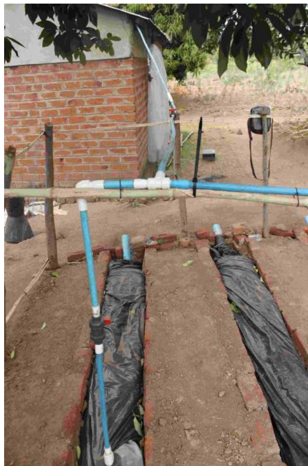
Figure 26: Biogas digesters with pipes leading to the storage bag and the kitchen.
