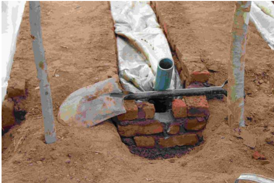
Figure 8: Newly made ending of a trench which allows the outlet of the pipe to be raised to the correct level.
