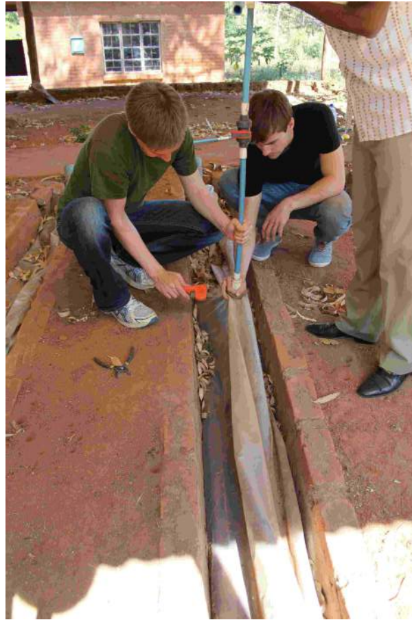
Figure 1: Dismantling of old digesters.
