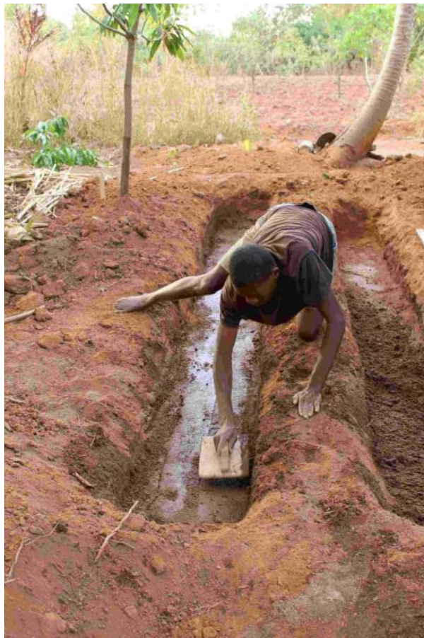
Figure 6: Cementing of trenches to ensure a flat ground level.
