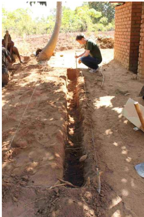
Figure 4: Measuring of trenches to ensure correct dimensions.
