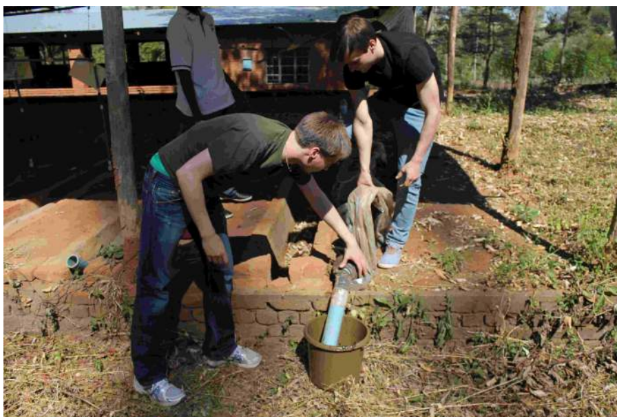
Figure 2: Emptying of slurry from an old digester.
