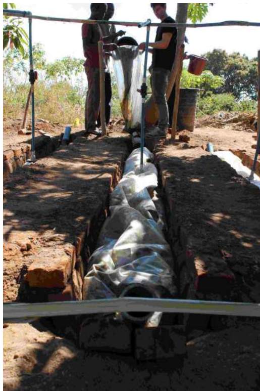
Figure 12: Filling of the tubes for the first time.
