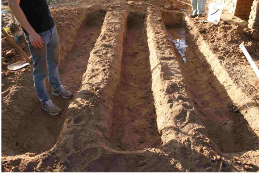
Figure 5: Dug out trenches ready to be cemented.
