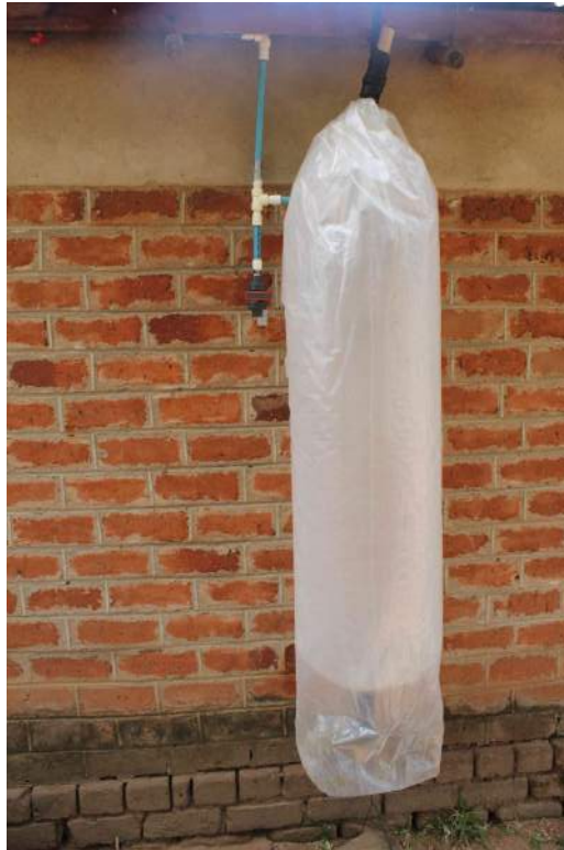
Figure 9: The storage bag was hung from the ceiling outside of the kitchen. When the picture was taken the storage bag contained around 200 litres of biogas.
