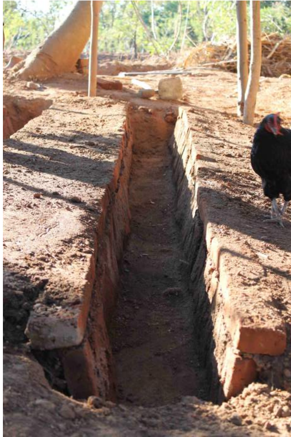
Figure 7: Trench with bricks on the side walls.
