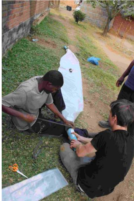
Figure 3: Fastening of PVC pipe to work as outlet of the newly made digester. Rubber bands from car tires is wrapped around in order to prevent leakage of slurry.
