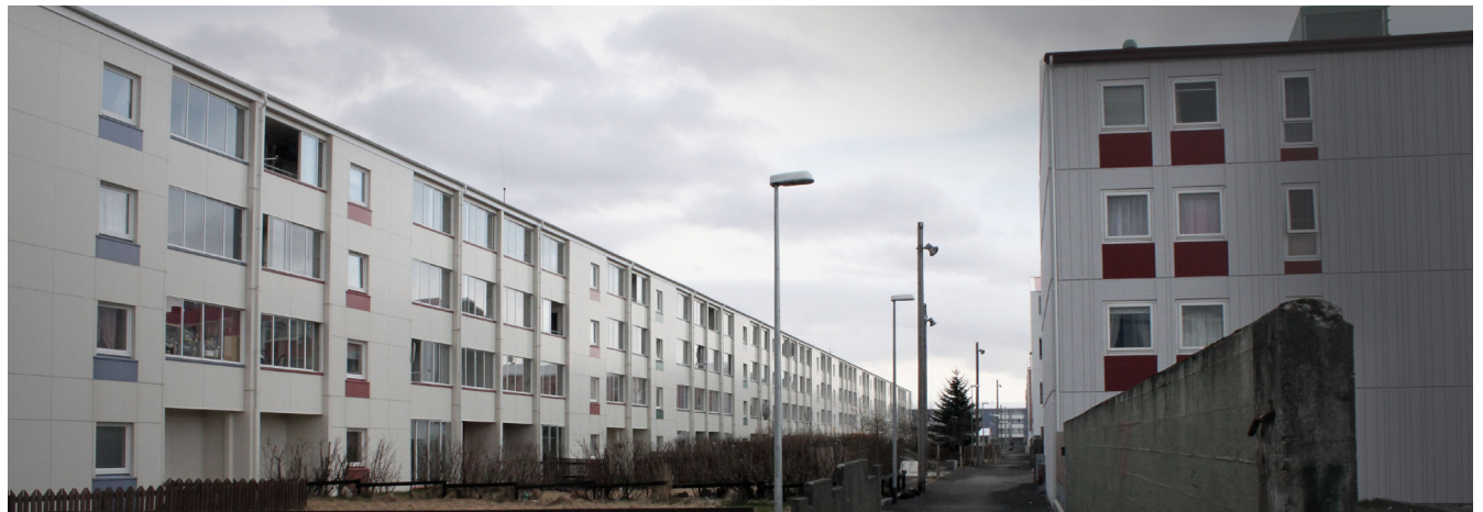
Figure 18. Buildings of Fannarfell,
