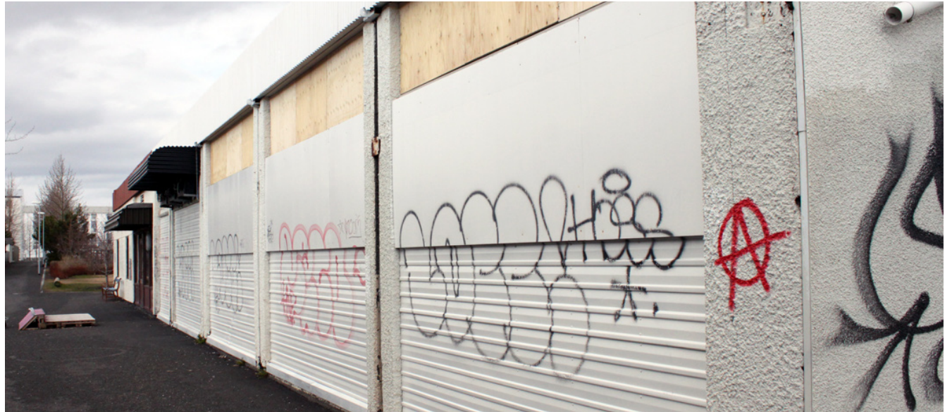
Figure 31. The backsides of businesses at Fellagarðar.
