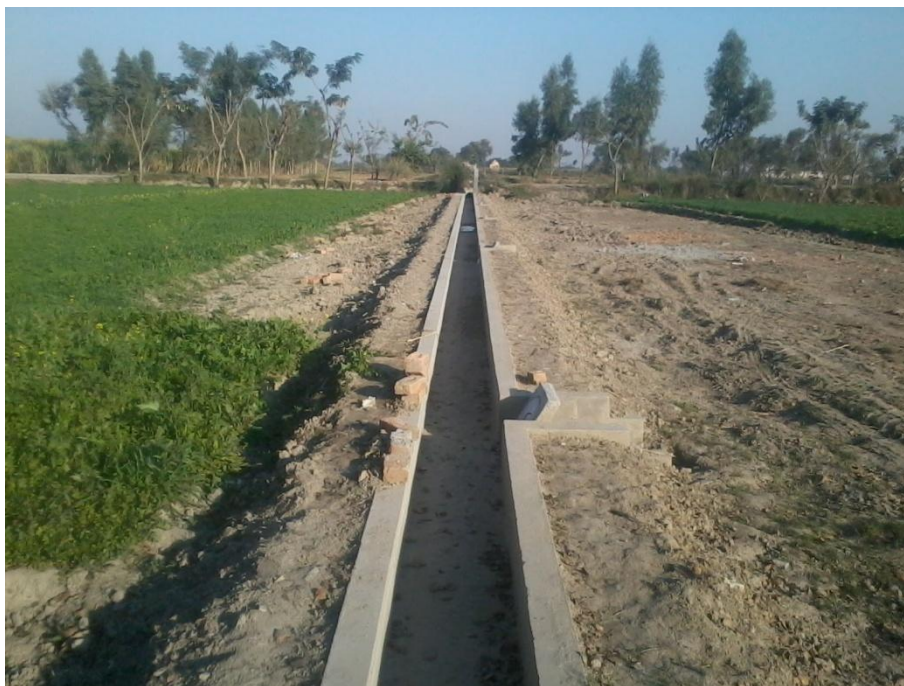
Figure 9: Watercourse lining with cemented bricks
