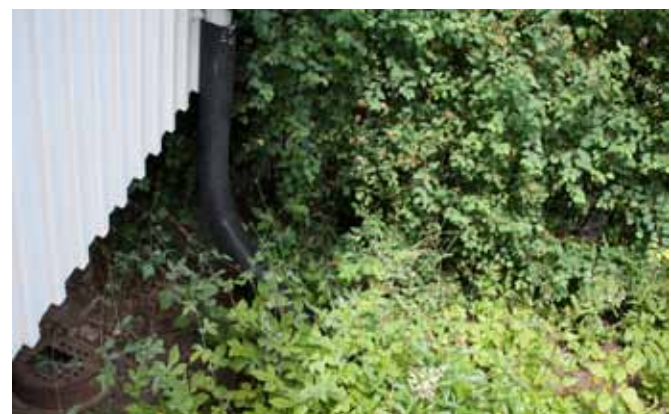
Figure 112. Author's own downspout located within Kvillebäcken's watershed that has been disconnected for a year without incident.
