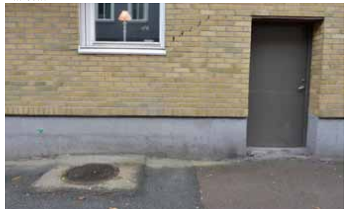
Figure 63. Settling pavement and cracked building in Brämaregården caused by the changed hydrology and increased load put on the soil below.
