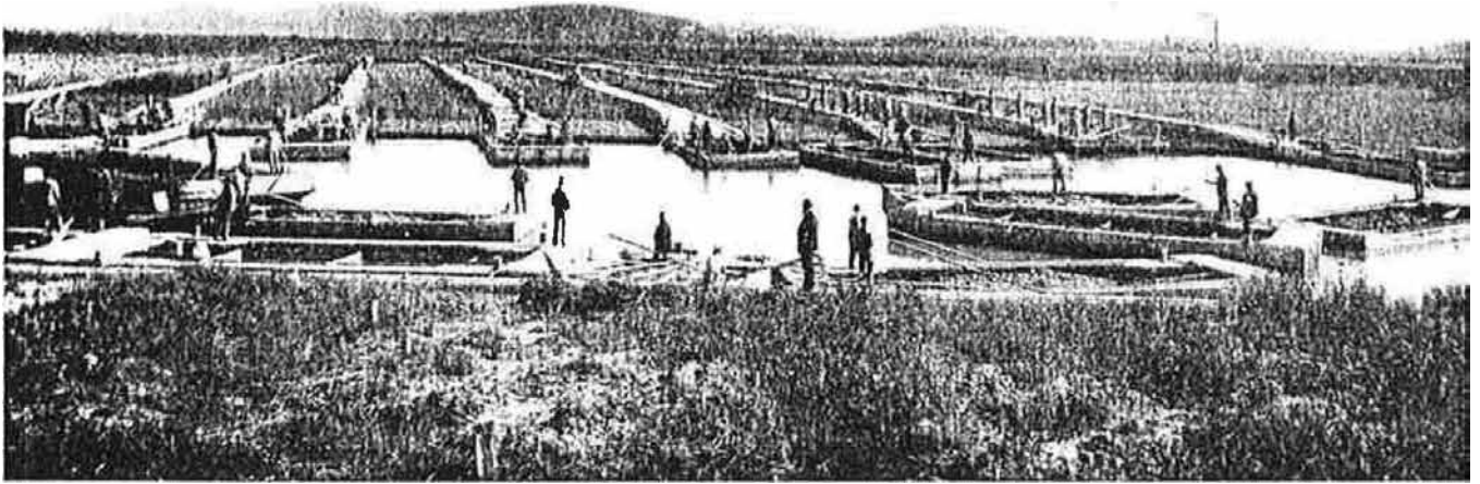
Figure 53. (Around 1850) Workers transported dredging material in wheel barrels pushed along boardwalks in order to fill the Tingstadsvass marshlands.
