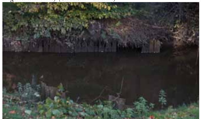
Figure 26. The stream banks are fortified with pilings 2011-10-1
