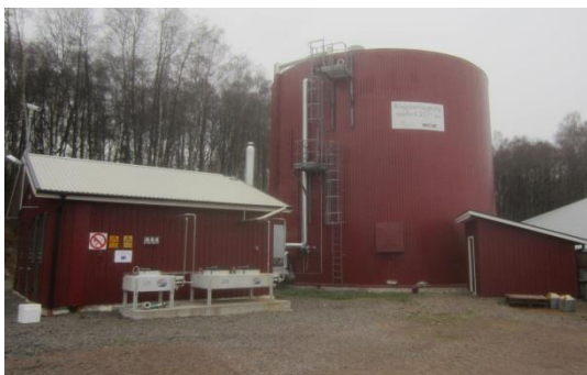
Figure 2: Högryd including digestion chamber and machine building
