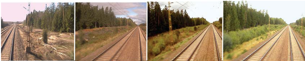
Figure 1. An example of a tree-cleared railroad, first picture after clearing was conducted, second picture one vegetation season after clearing, third picture two vegetation seasons after clearance, and the fourth picture shows the vegetation after three vegetation seasons. Photos from a STRIX-movie, provided by the Swedish Transport Administration.
