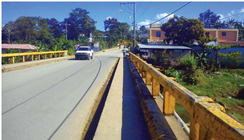
Figure 78: Current bridge. The pedestrian lane is very narrow and general accessibility is deficient. Miches, 2012
