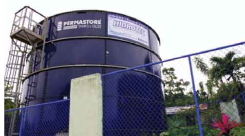
Figure 45: Water cistern. Miches, 2012
