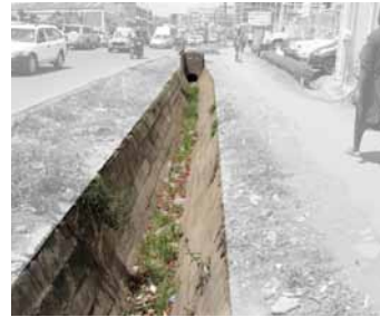
Hard trenches are collecting and leading water in Nairobi. They separate the road from the pavement.
