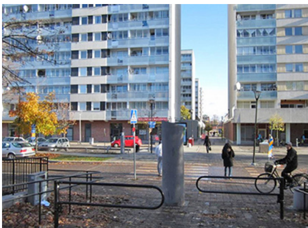
Apartment buildings of Malmvågen.
