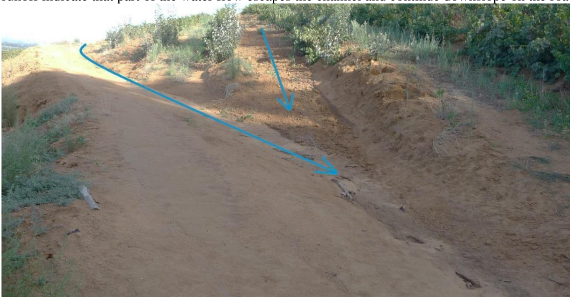
Figure 34 Water released by the waterway, seen in figure 29, is transported on a gentle slope cause rill erosion when uniting runoff from block 309. Eventually, diverted to the forest by an earthen channel.
