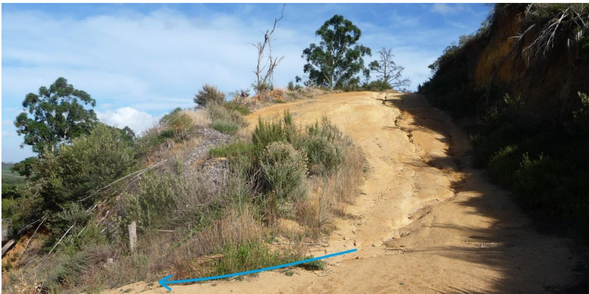
Figure 42 Water flow eventually reach an area of natural vegetation where the speed of water is slowed down by natural vegetation and safely transported down the steep slope, to the left, not causing any further damages.
