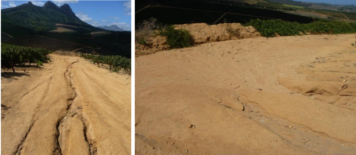
Figure 43 Left: Rill erosion occurring on the road in the middle of block 512. Right: At the cross-road runoff is trapped by an earthen wall which slow down the speed and force of water flow significantly.
