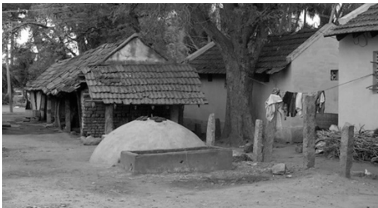
The white concrete sphere is a tank that produces biogas.
