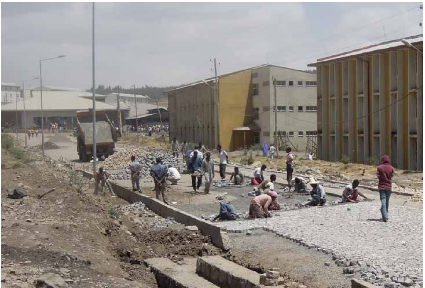
The area is still under construction.
