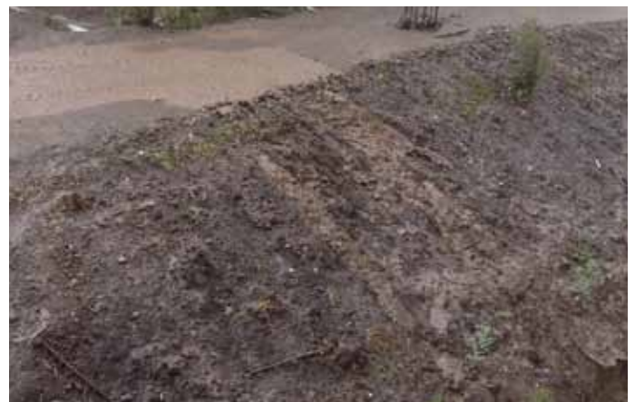
The ground materials are swept away with the water runoff.
