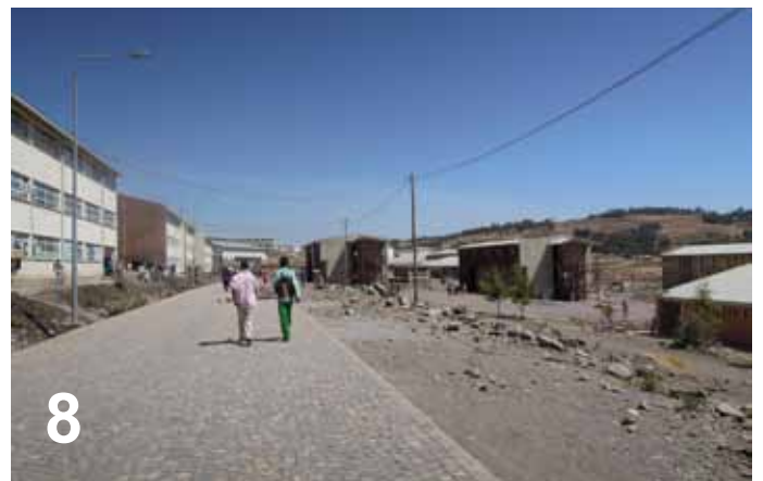
The road alongside the administration area with a big open space on the right hand side.
