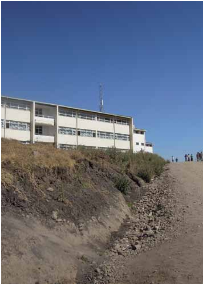
The ground is very steep towards the male residential area.
