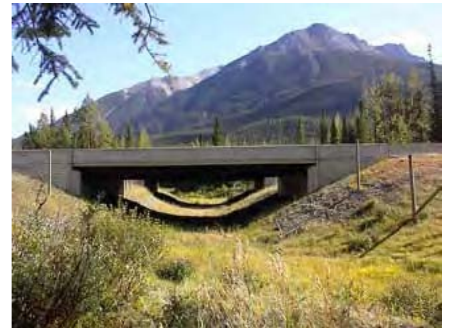
Figure 245: An underpass keeps the green link unbroken and makes it possible for species of animals and plants to spread without disruption. Source: TransWild Alliance 2012.
