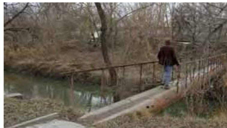
Figure 210: Pedestrian bridge constructed on pipes.
