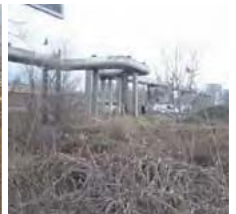
Figure 213: Gas-pipes crossing the river.
