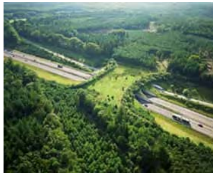
Figure 247: An ecoduct is another solution for avoiding the barrier-effect from a road network. This example is taken from: Urbanity.es 2008.
