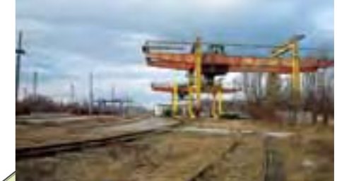
Figure 97: The railway creates a barrier and divides the city in two parts. Photo by: Johanna Hagberg
