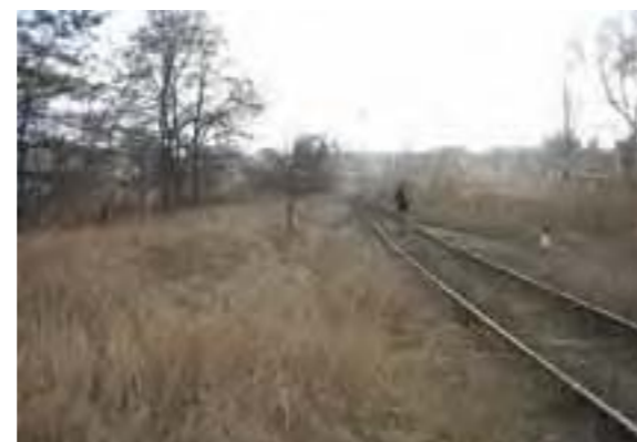
Figure 219: There are very few cross-points for pedestrians over the railway.
