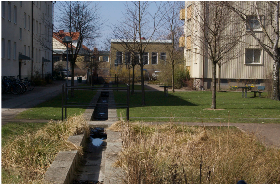
Cement and sandstone canal with grass-covered overflow area at Augustenborg. Photo by Scott Wahl taken April 2009
