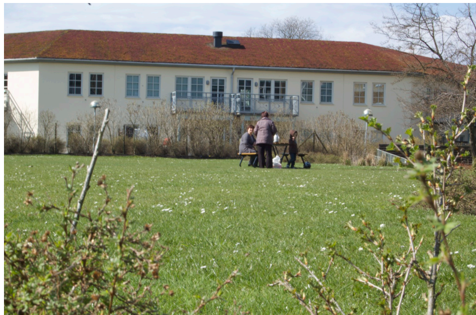
Green roof at Augustenborg. Photo by Scott Wahl taken April 2009
