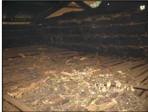
Figure 3. Empty storage attic where maize is stored on the floor.
