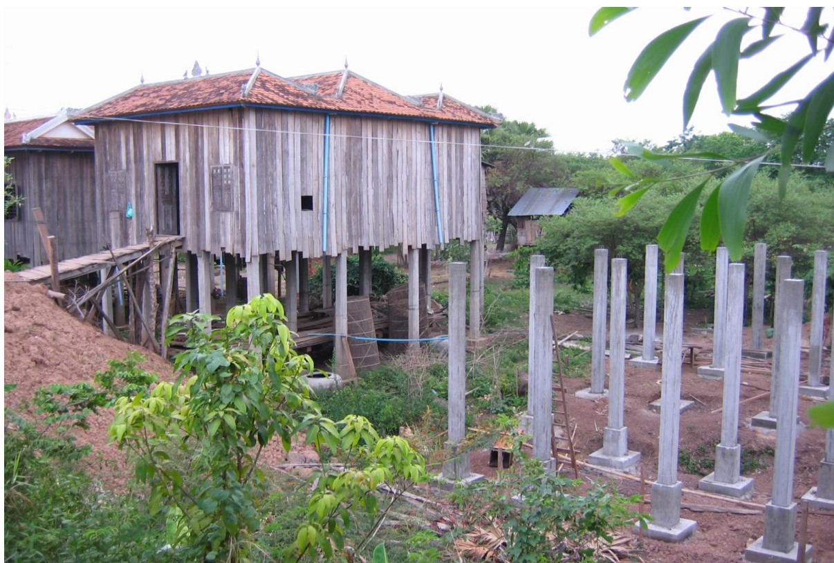
Pict. 6.1 The concrete poles, and the house with the ramp leading to the elevated road
