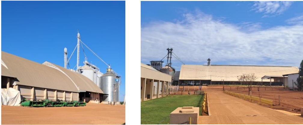
Figure 13. Soybean and corn storage silos, Sorriso, Mato Grosso, Brazil - a first aggregation point: (a) storage silos and warehouse; (b) grain aggregation facility, complete with weighbridge. Photograph courtesy of Júlia F. Viotto, 2026.
