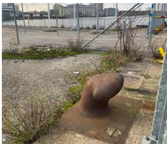
Fig. 36: Mooring bollard and fenced areas
