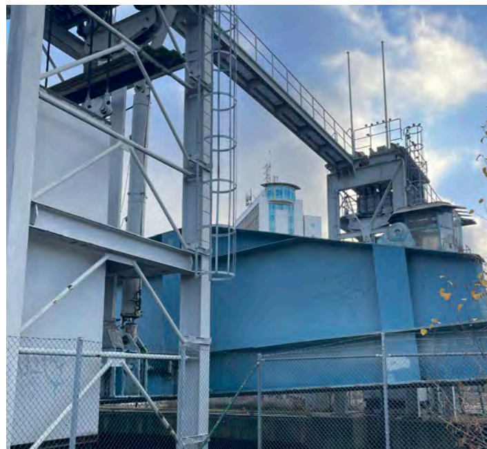
Fig. 7: Abandoned industrial sites are interesting for development
