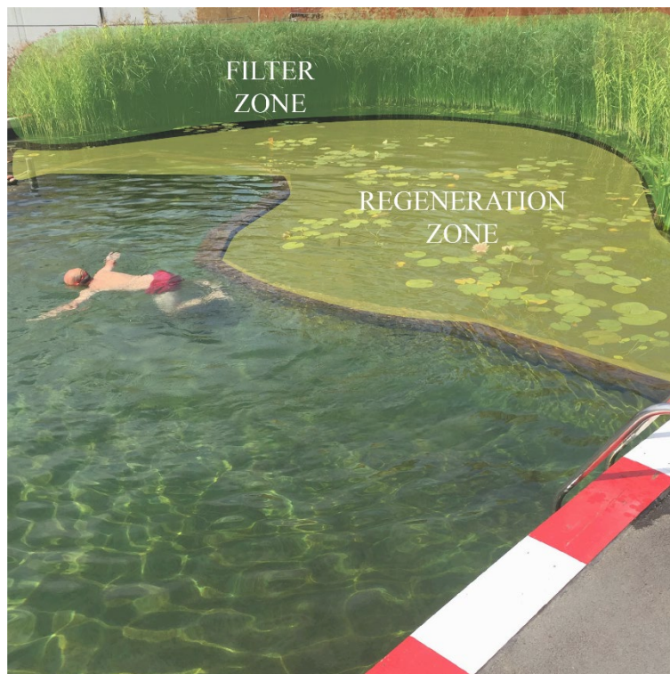
Figure 22. Picture of King's Cross's filter and regeneration zone highlighting the two zone's high in the landscape (BD Landscape Architects, 2022); modified by author.
