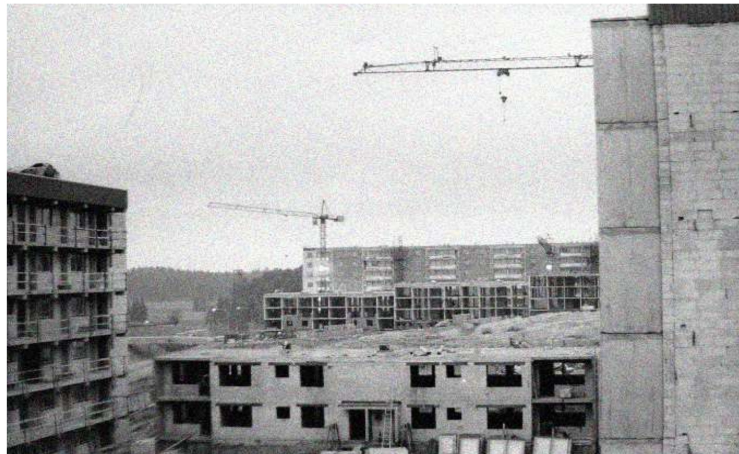
Figure 3.1. Archive image of the construction of Tensta, Stockholm (Svenskabostäder 1967) (CC BY-NC-ND 2.0).
