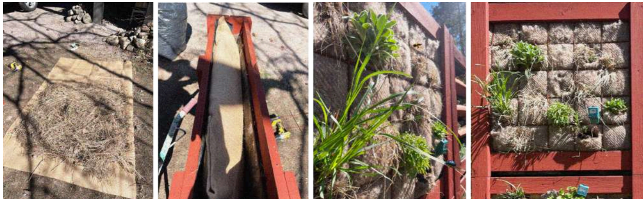
Figure 6.41-44. Construction images module 01, April 2026.
