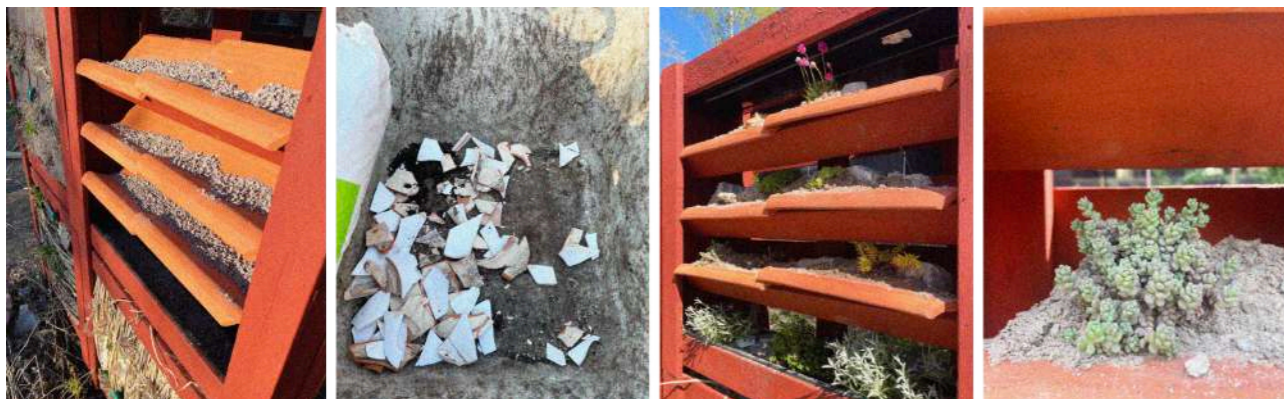
Figure 6.45-48. Construction images module 02, April 2026.
