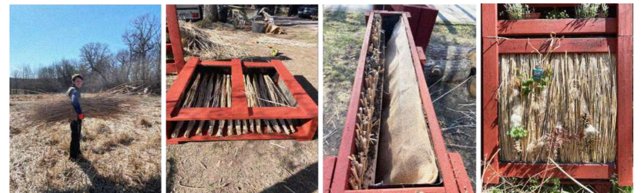
Figure 6.53-56. Construction images module 04, April 2026.
