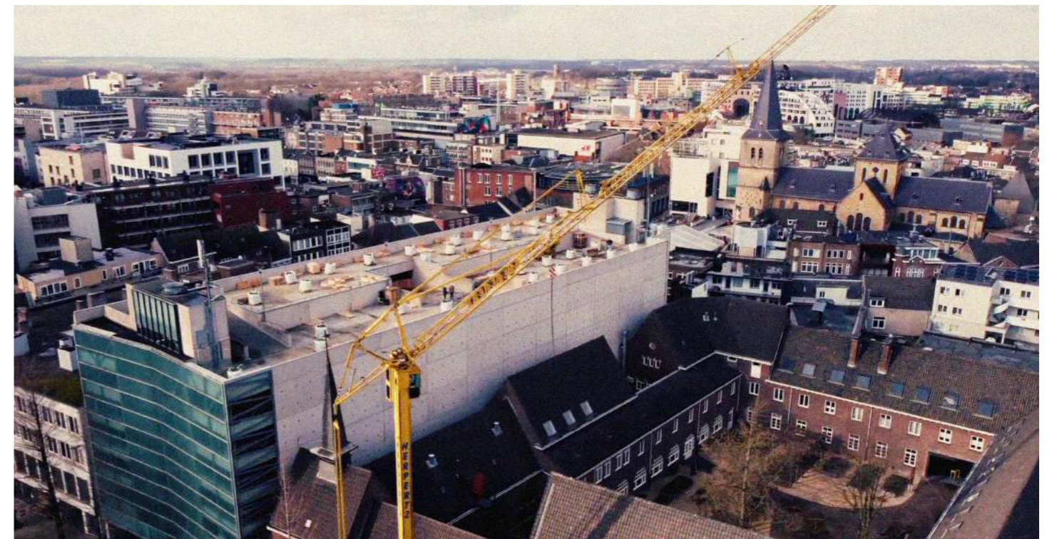
Figure 6.5. Heerlen Rooftop Project. (Schunck 2022) (CC BY 4.0).
