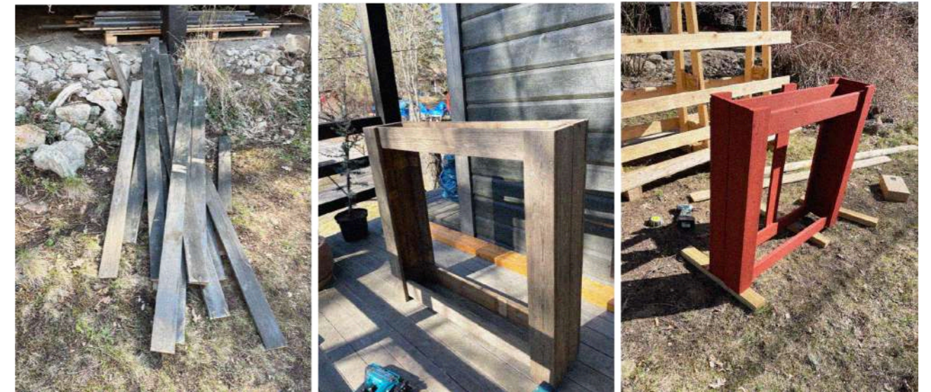
Figure 6.38-40. Construction images of the wooden framework for the base-modules, April 2026.
