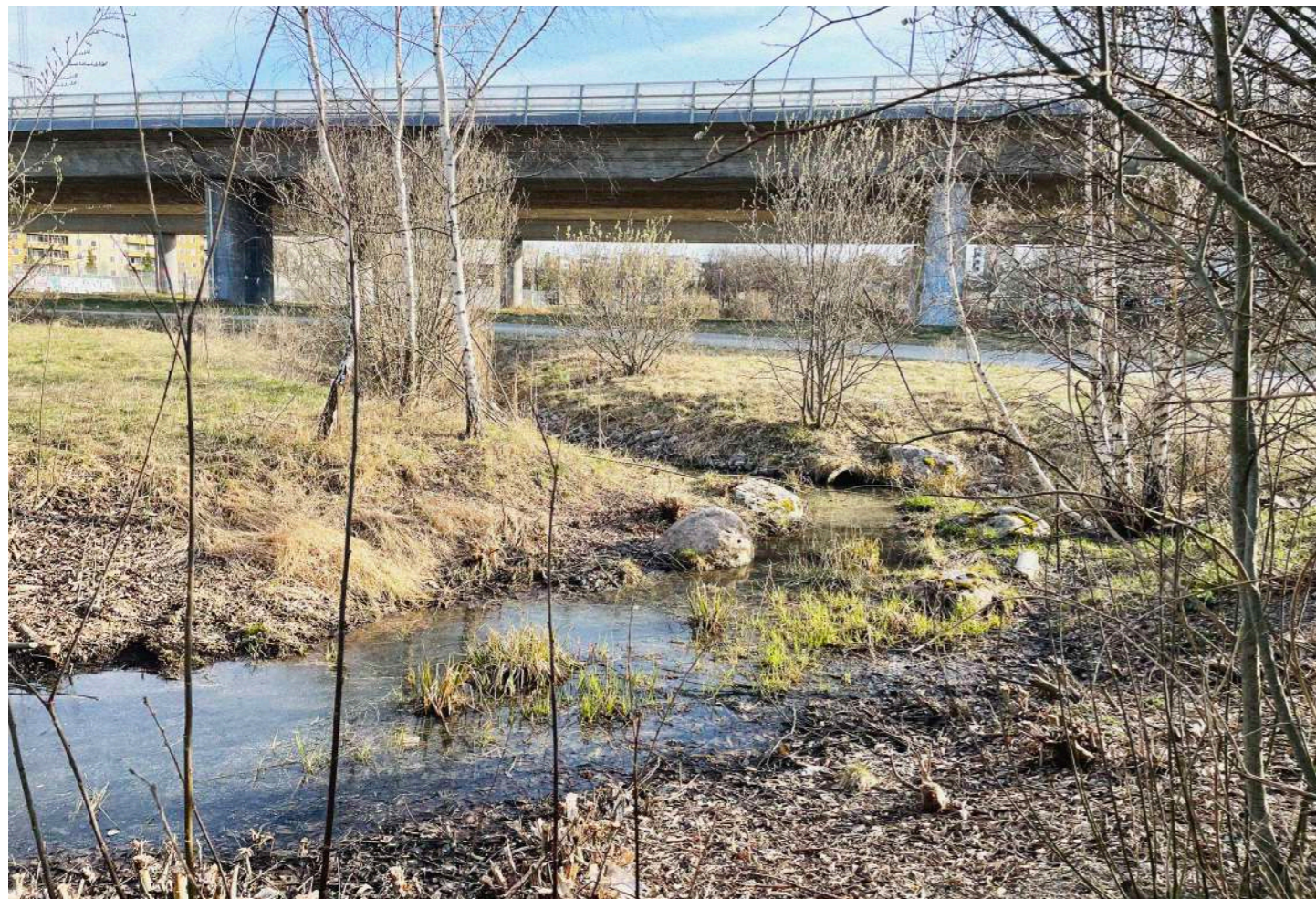
Figure 3.10-13. Views from Järfället towards Tensta illustrating the hard edge between nature and the city. High concrete façades reflect the noise from the E18 highway, reinforcing both a visual and acoustic barrier between the urban fabric and the surrounding natural landscape, April 2026.
