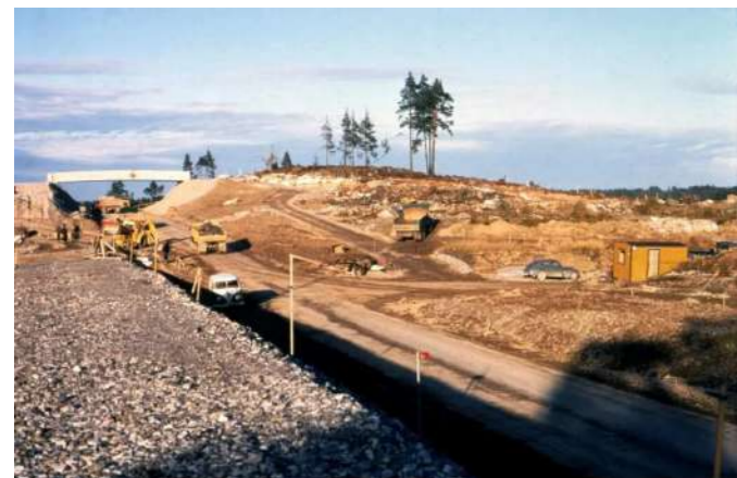
Figure 5.3. Construction of Tenstraket (Kallbergberg 1968) (CC BY 4.0)
