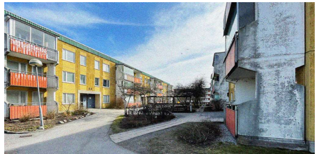
Figure 3.4-6. Occasional encounters with construction waste and scaffolding along façades in MHP area Tensta, Stockholm indicate ongoing renovation practices. However, many façades show clear aging signs and need for renewal, February 2026.
