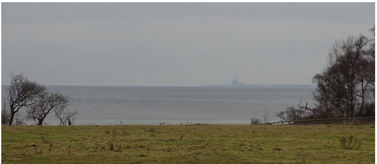
Figure 8. Photograph of the pasture from a viewpoint in Lomma. The power plant is viewed more closely. [photograph by the author, 2026-01-26]
