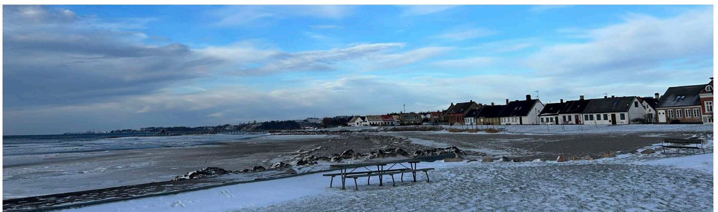
Fig 61: Borstahusen's coastline. One can see how close the buildings are to the sea (Jönsson Karlsson, 2026)
