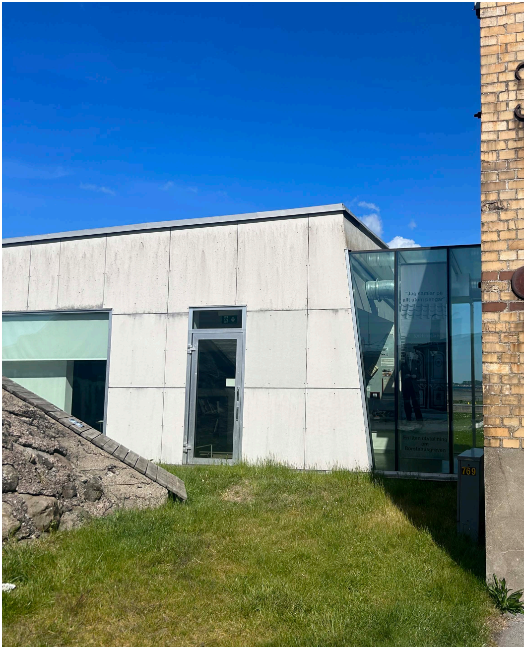
Fig 49: The old pump house serves today as an art gallery and museum, and has been connected to the new modern restaurant building (Jönsson Karlsson, 2025)
