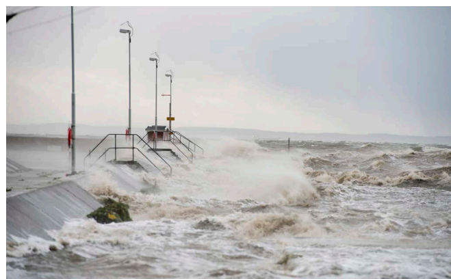
Fig 63: The sea washes over the long concrete pier Cement in Borstahusen during the storm Sven. (AT Foto, 2013)
