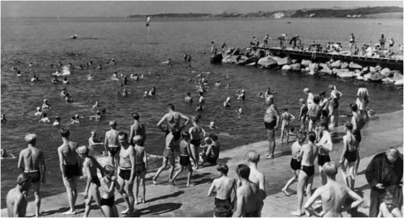
Fig 46: The harbour after the reinforcement with cement. Lots of people swimming and jumping into the water (Landskrona museum, 1947)
