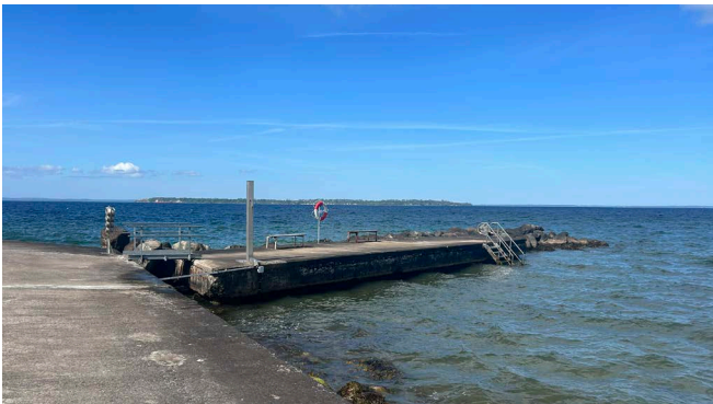
Fig 65: Cement arm/pier stretching out from the harbour (Jönsson Karlsson, 2025)
