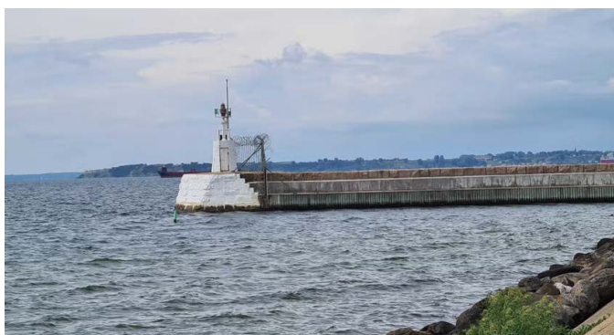
Fig 8: Groyne/reinforced harbour (Ermeland, Matilda, 2021)
