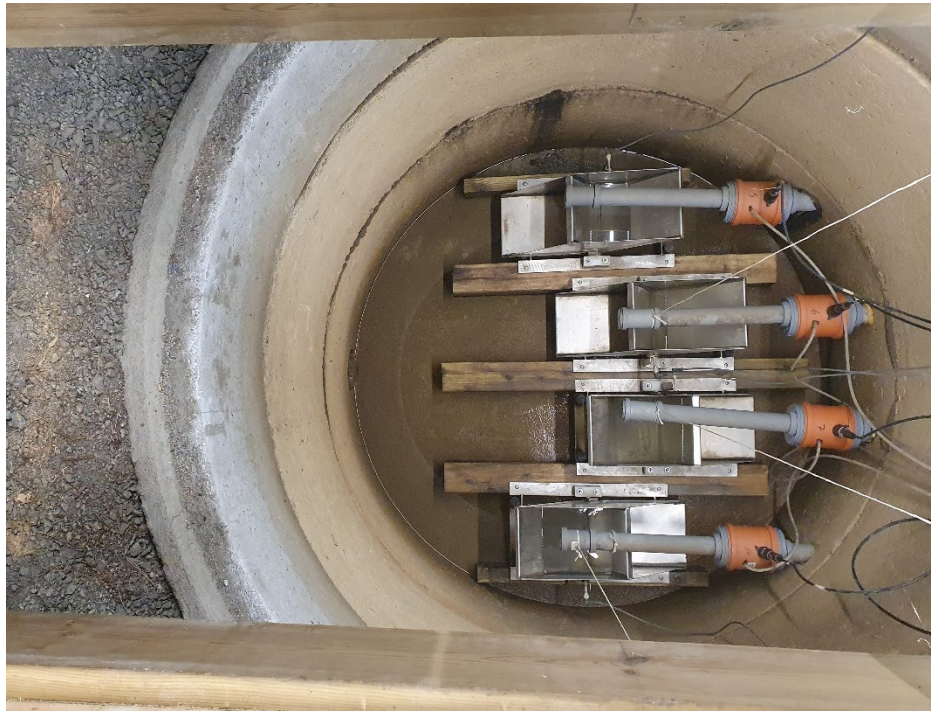
Figure 4. The two-sided tipping buckets from four of the drainage pipes of the plots in the field trial. Photo: Linnea Berggren Sjögård
