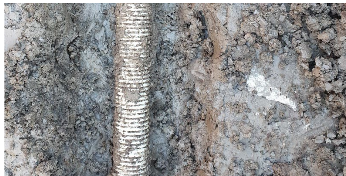
Figure 10. Plot 6, to the right of the pipe there is a flat, hard, whitish surface at the same depth as the drainage pipe, approximately 1 m. Photo: Linnea Berggren Sjögård
