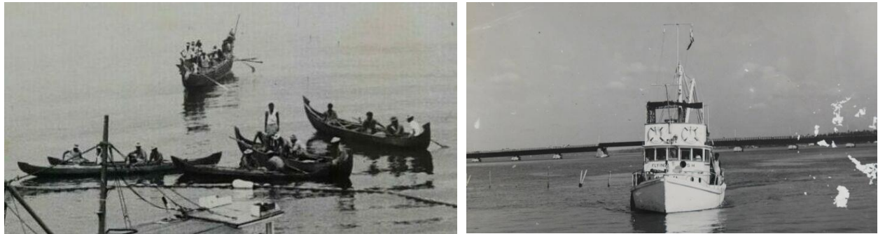
Figure 28: Country crafts like dugout canoes (made of single logs) were used for fishing until the mid-twentieth century. These types of boats are still in use in Kerala (left). Flying Fish, a trawling boat made as part of the INP. The metallic structure to haul the net can be seen behind the cabin (right). (Image: NIFPHATT, Ernakulam, 2023)
