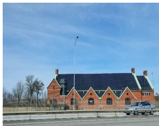
Figur 3 Rosendals pumpstation. (Jonsson E, 2024)
