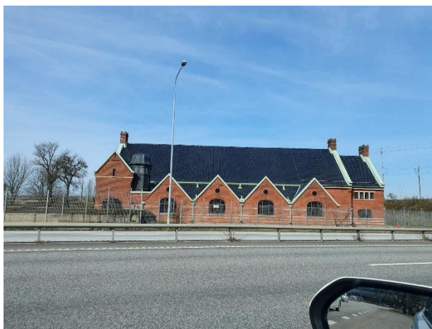
Figur 19 Rosendals pumpstation. Jonsson, E (2024)
