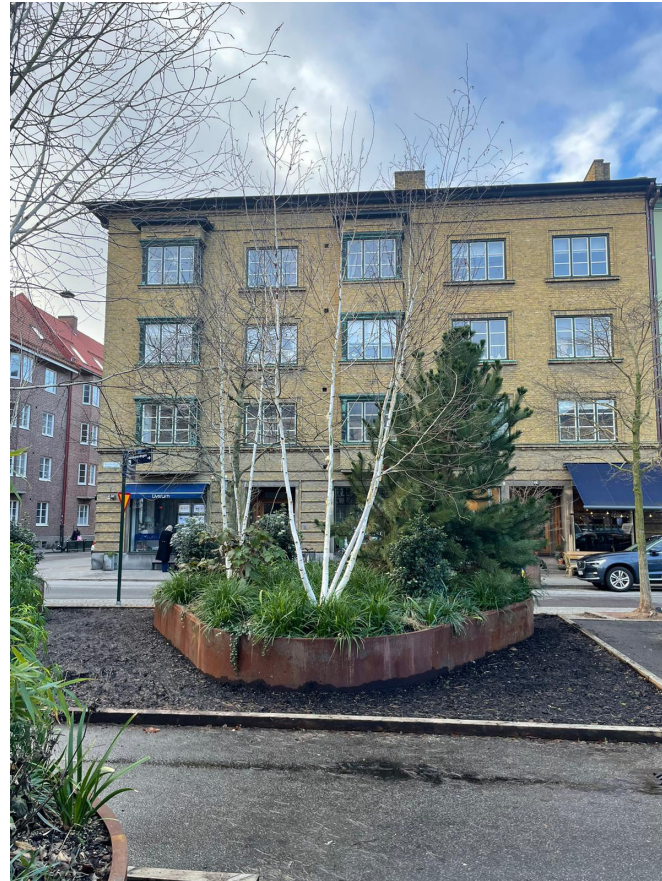
Figure 19. A temporary planting container constructed with corten steel. Located in Davidshallstorg, Malmö.
