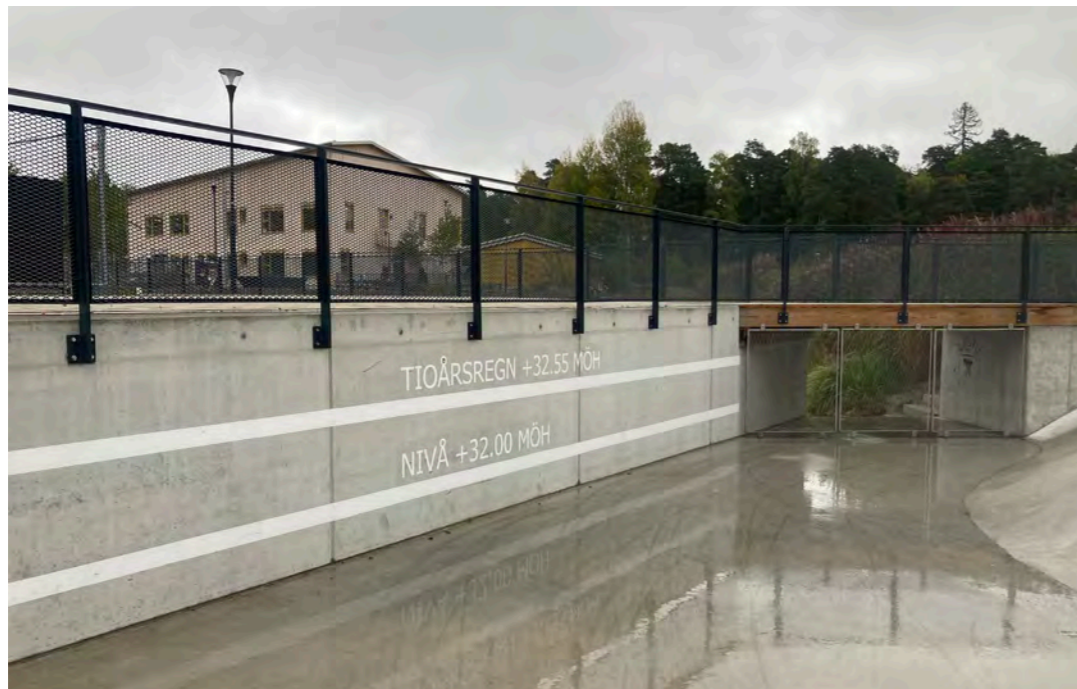
Fig. 37. The multifunctional retention storage and its overflow connection to the pond. On the wall are markings for different storm event water levels, Basin , Flemming Pedersen, 2023.
