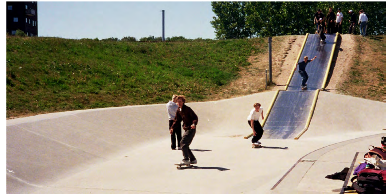
Figure 32. In Rabalderparken, Denmark, recreational values have been integrated into a large-scale stormwater facility, Rabalderparken, Emmilou Holmgren, 2023.
