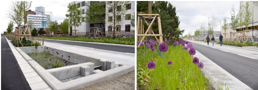
Figure 17 and 18. Neptunigatan Malmö, biophilic street with storm water management and separation between cars and other users. Photo by Edge 2019.
