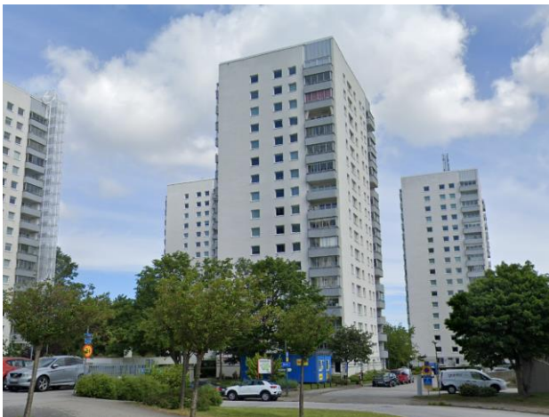
Figure 39. Image of High-Rise Tower Blocks in Höegaholm, Almvik. One of the few really tall ones in Malmö Source: Google Maps, 2024
