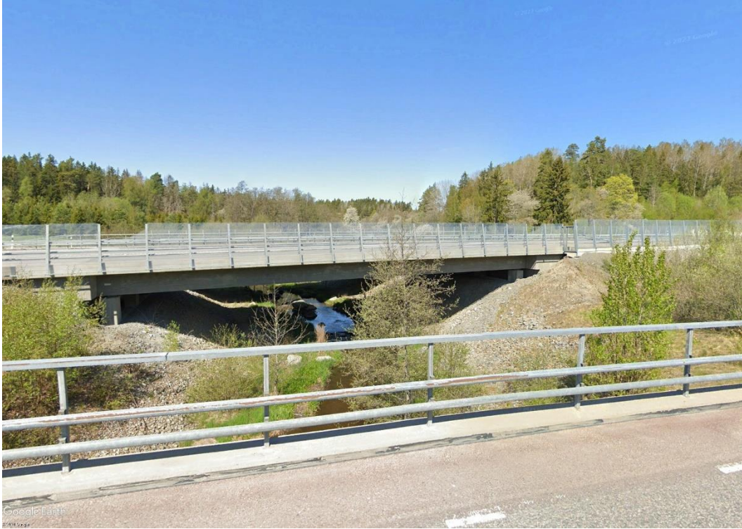
Figure 17 Underpass, Road 73 (Google Earth; Street View)
