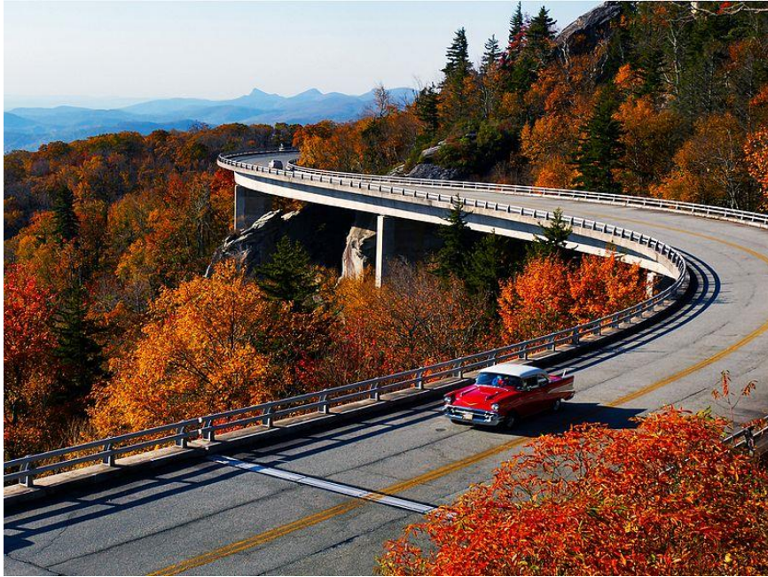
Figure 7 Example of a viaduct (Mbugbey)
