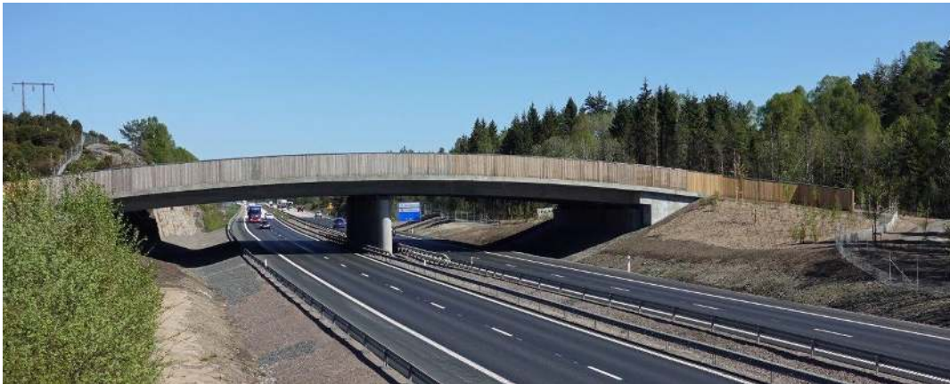
Figure 9 View from E6 towards the north. Newly built ecoduct, May 2018
