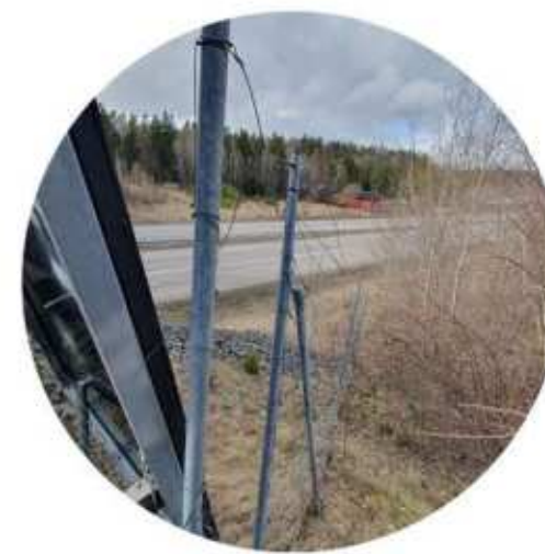
Figure 32 Broken fencing
