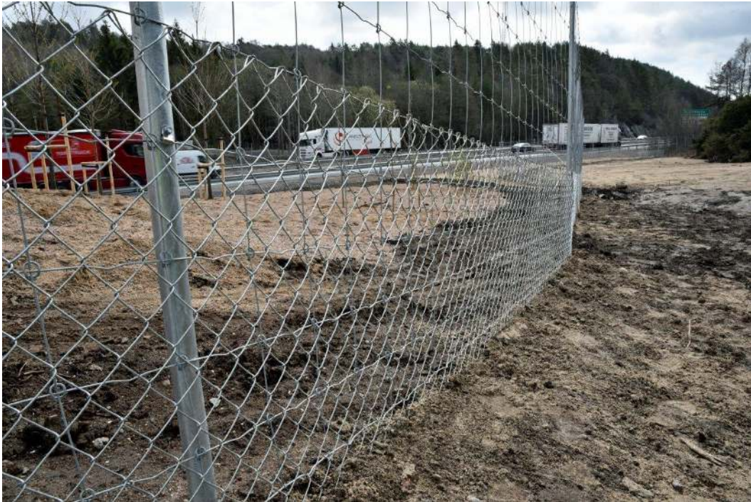
Figure 11 Fencing buried in the ground to prevent wildlife from digging their way out to the road (Mats Lindqvist)
