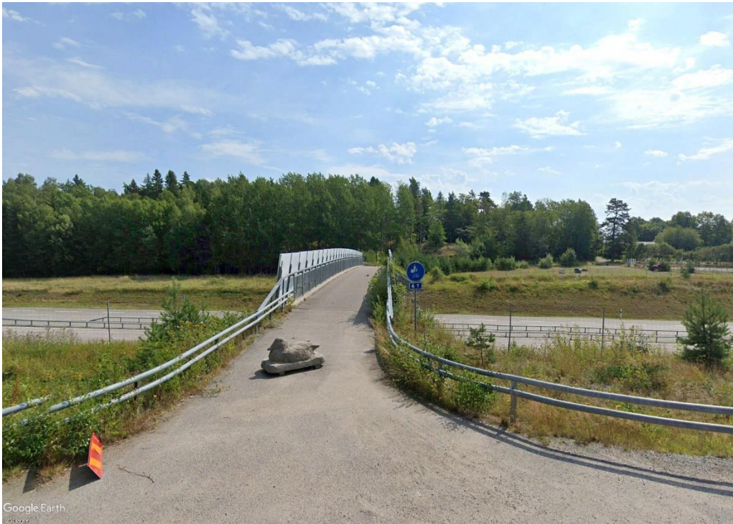
Figure 16 Pedestrian bridge on Road 73 (Google Earth; Street View)
