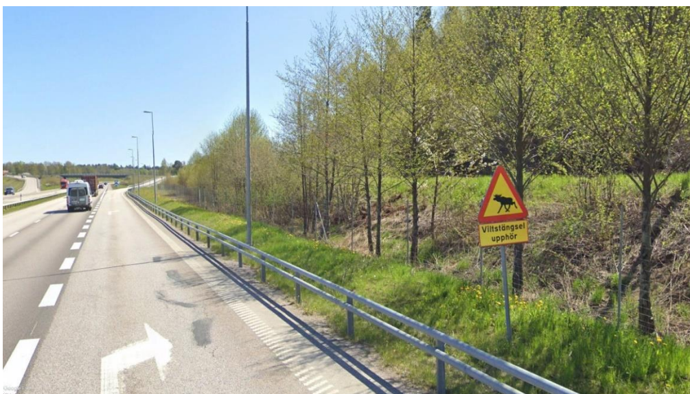
Figure 19 Fencing ends (Google Street View)
