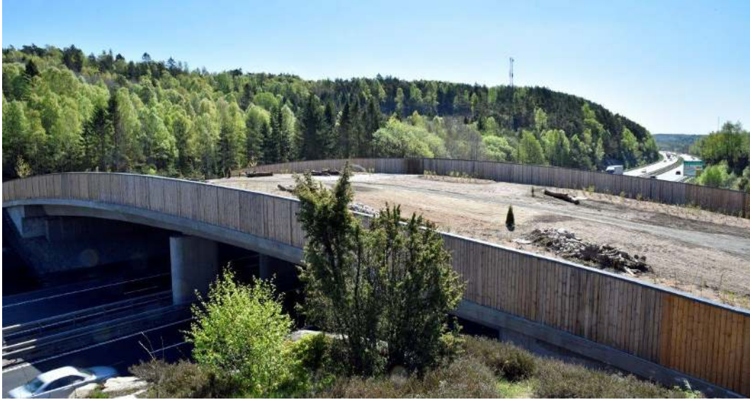
Figure 10 West to the east view of the ecoduct with newly planted vegetation and various small biotopes, May 2018 (Mats Lindqvist)
