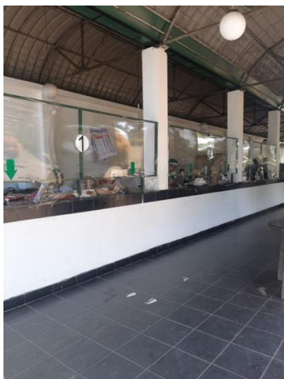
Figure 15. Structure of the food outlet (Source: Author)
