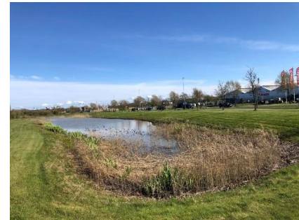
Figure 7. Flygstaden Stormwater Pond Halmstad Municipality (photo: Mikael Brocki).
