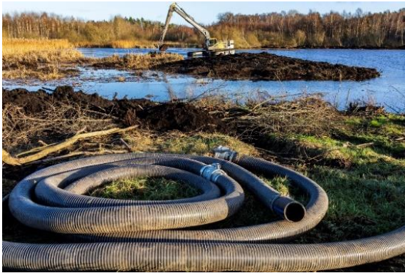
Figure 18. UW-Dredging (photo: Peter Johnsson).
