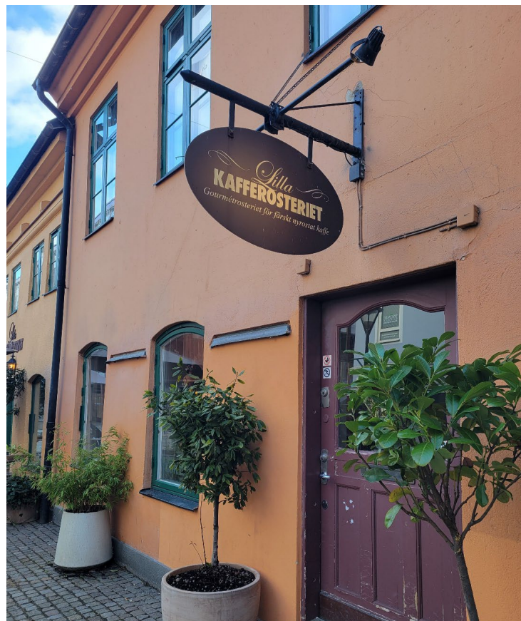
Figure 15: Lilla Kafferosteriet's "old yellow house". Lilla Kafferosteriet's original roastery location was in an historic 15th century house in Malmö's Gamlastan (Old Town). The building still houses the brand's coffee shop and architecturally connects the brand to Malmö's heritage.
