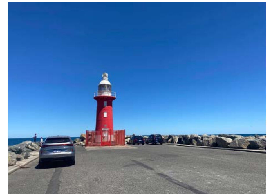
Figure 51: The red lighthouse at the finish of the mole that can be seen from a distance.
