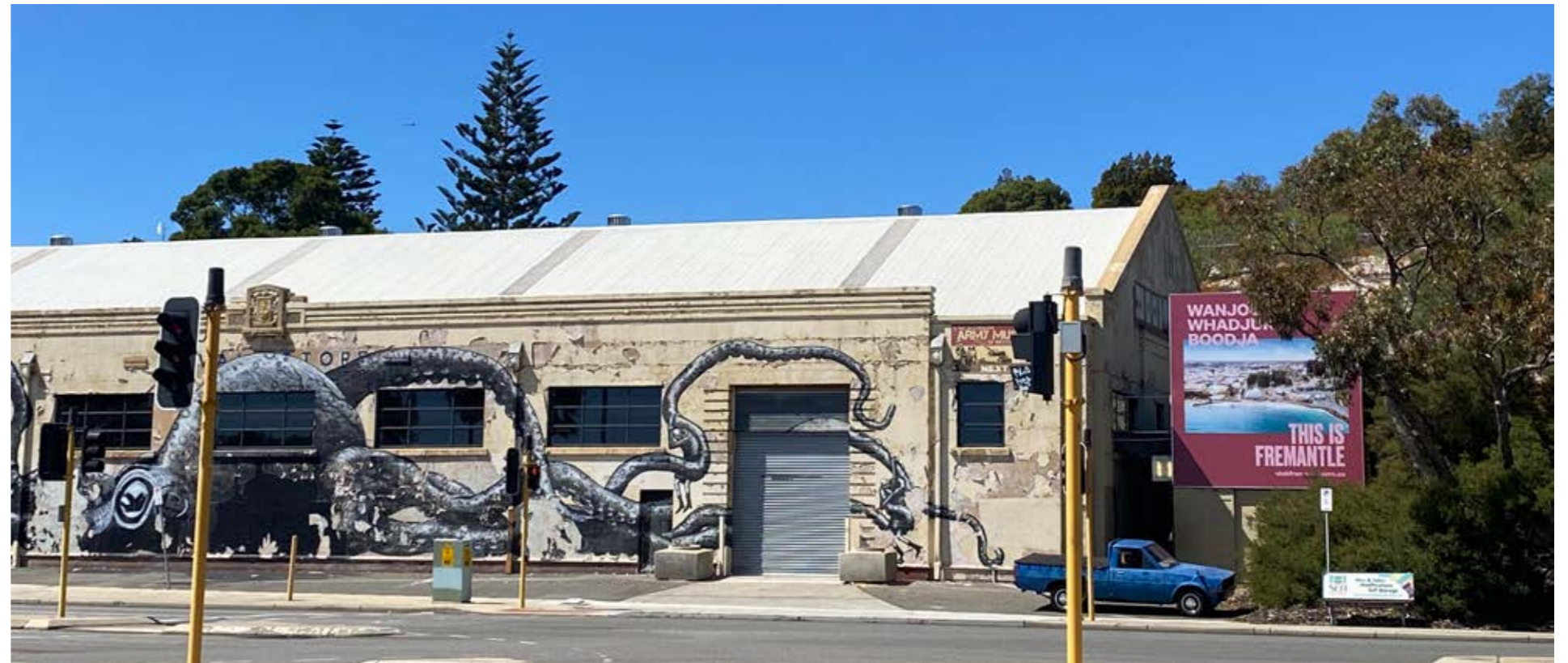
Figure 8: Graffiti on building in Fremantle, which is recurring in Fremantle.
