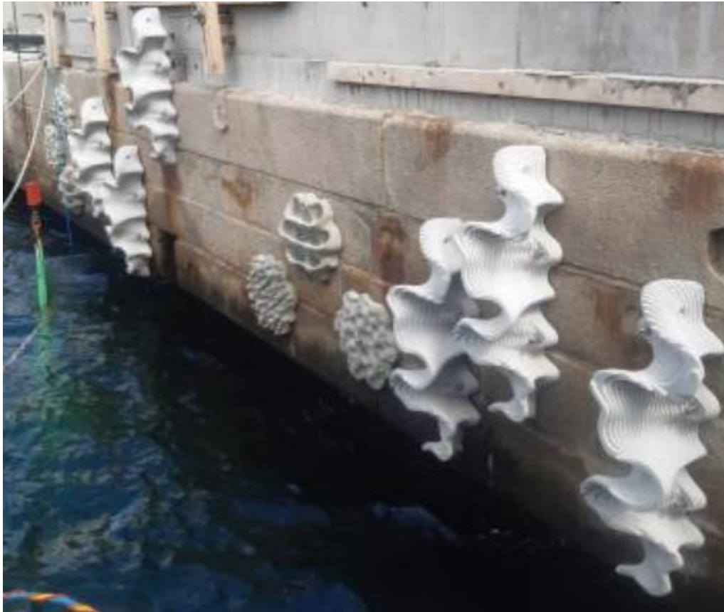
Figure 3. The above water section of the living seawall. Photo credit (Bertilsson Vuksan 2022).
