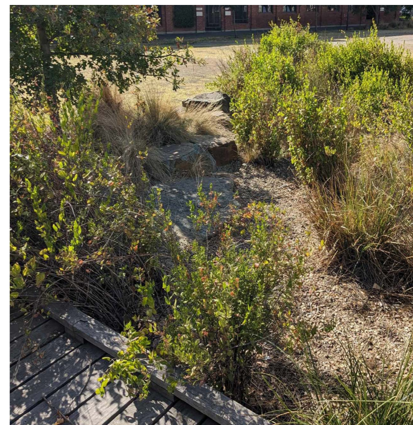
Figure 62 showing a photo of a swale in Kirrip park, planted with native vegetation, and a wooden bridge for crossing.
