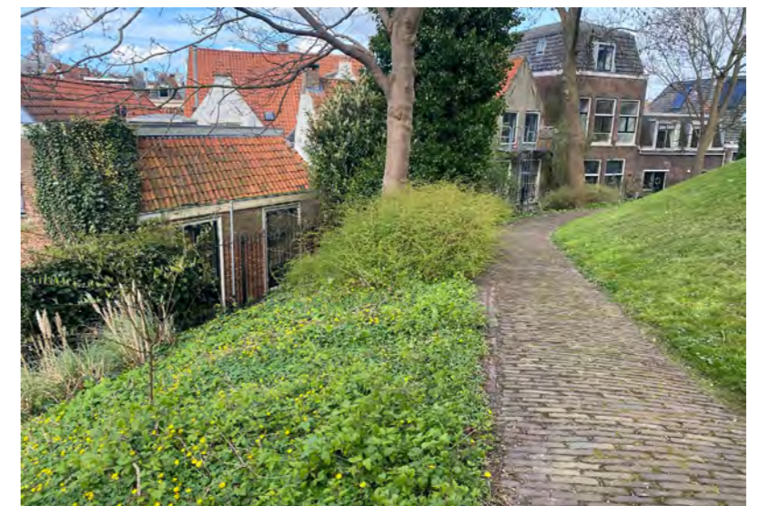
Figure 102: Running bond with similar colours that used in the design , Leiden , the Netherlands © Kittima Ritthichot (2023).
