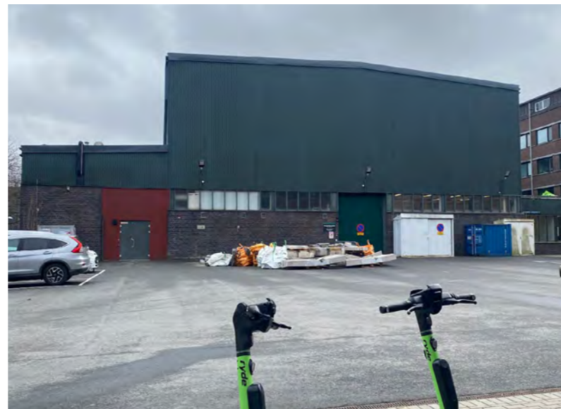
Figure 49: Entrance port for facility workers and cargo port, some part of the open space is used for material experiments and fraternity activities © Kittima Ritthichot (2024).
