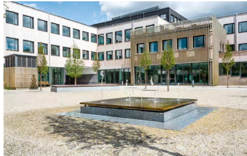
Figure 85: The water fountain that invites users users to experience the element as they transion through the courtyard © Bo Gyllander (n.d.e).
