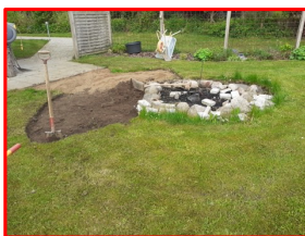
A bond-fireplace (work in progress)
