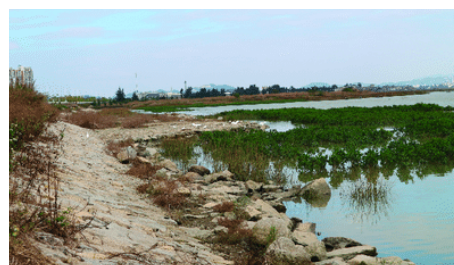
Fig. 22. Seawall and marshes (Lu et al. 2018:17).
