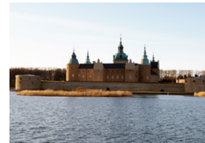
Fig. 120. Kalmar slott can be seen from the street at Barlastholmen.
