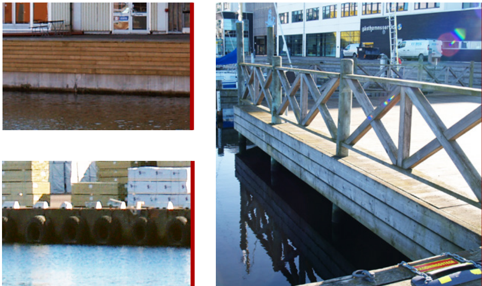
Fig. 29, 30 & 31. Hard structures; Concrete walls clad with timber or tiers.
