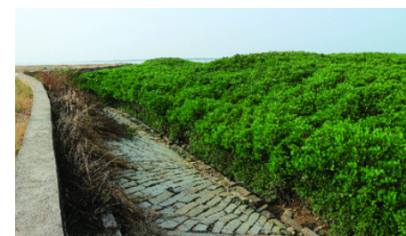
Fig. 23. Seawall and marshes (Lu et al. 2018:17).
