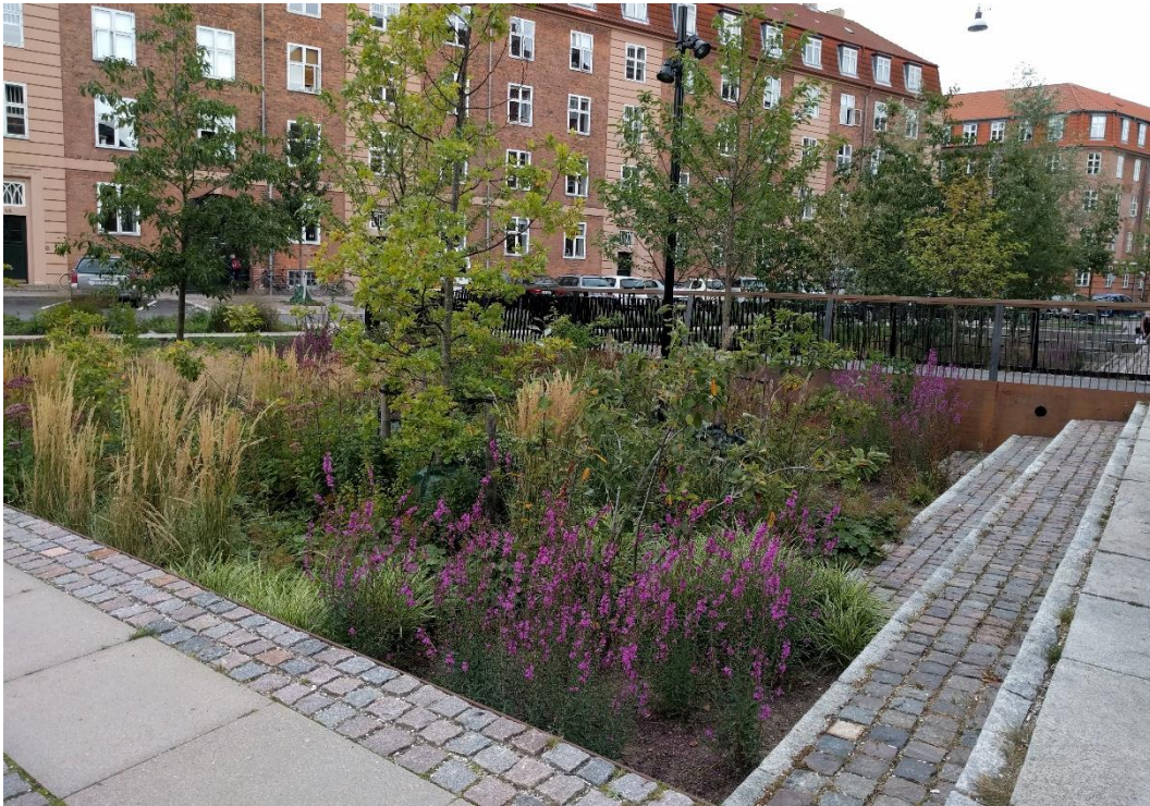
Figure 7. Water retention and seating at Tåsinge Plads in Copenhagen, Denmark (Gudrun Rabenius 2016).
