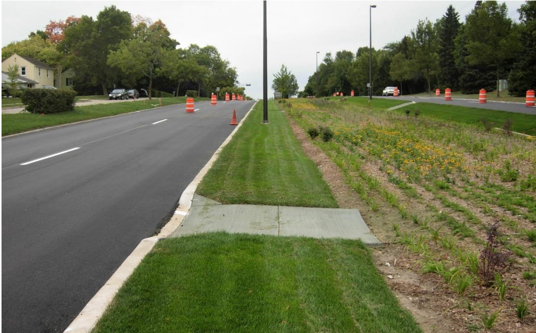
Figure 8. Bioswale and bioretention area in Greendale, Wisconsin, USA (Aaron Volkening 2009). (CC BY 2.0)
