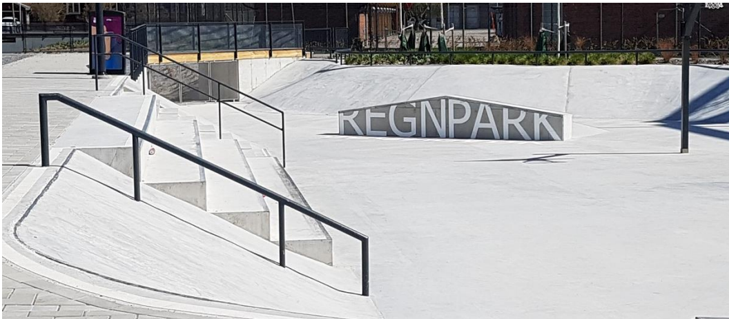
Figure 16. Activity area designed to handle planned flooding in Elsa Eschelsson's park in Rosendal, Uppsala, Sweden. The text reads "regnpark", i.e. rain park.
