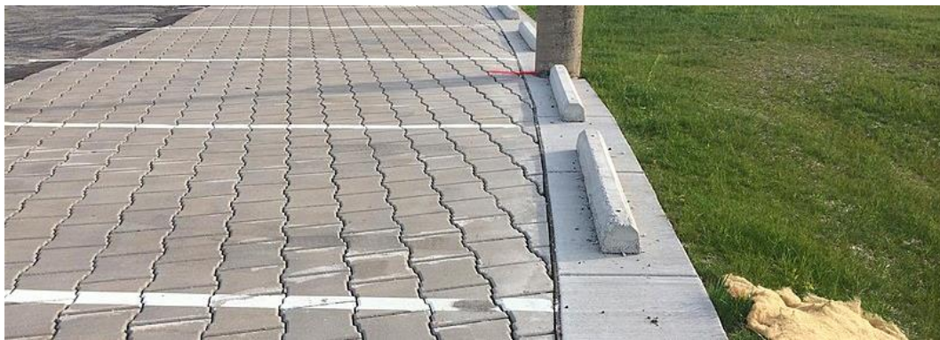
Figure 2. Permeable pavement at Greenfield City Hall, Greenfield, Wisconsin, USA (Aaron Volkening 2014). (CC BY 2.0)
