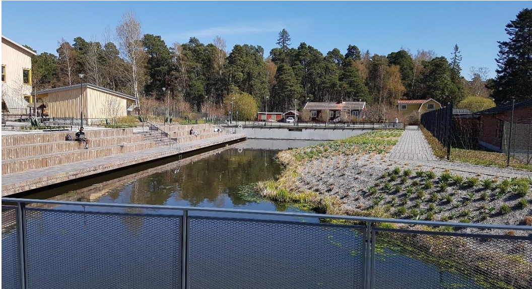
Figure 15. Stormwater pond for planned flooding at Elsa Eschelsson's park in Rosendal, Uppsala, Sweden.
