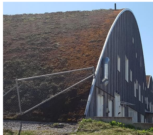
Figure 4. Green roof at USIF Arena in Rosendal, Uppsala, Sweden.
