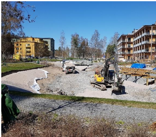
Figure 17. Construction at Carlshage park in Rosendal, Uppsala, Sweden.
