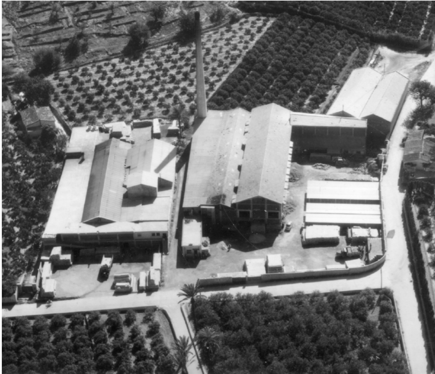
Fig. 20. The factory building to the right is the only one still in use. "Anticfang" still use the same techniques for their ceramic production as in the factory's heyday. Aerial photo from 1967. Unknown photographer.
