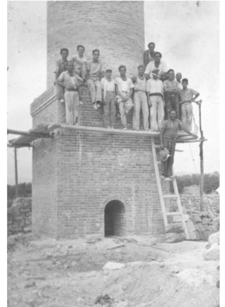
Fig. 17. Construction of the chimneys. Photo by: Javier Garrido
