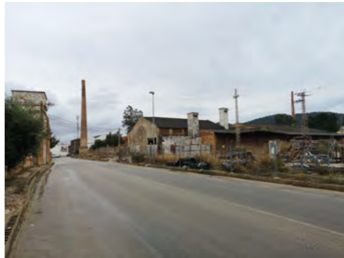
6. Fenced off material depot on the right.
