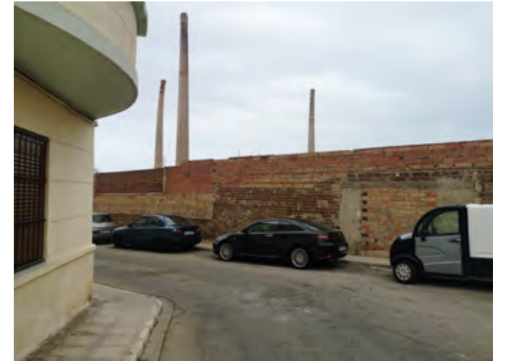
4. A peculiar view to see the chimneys reaching up behind the wall. The patchwork of the wall tells a story of many adaptations made in the past.
