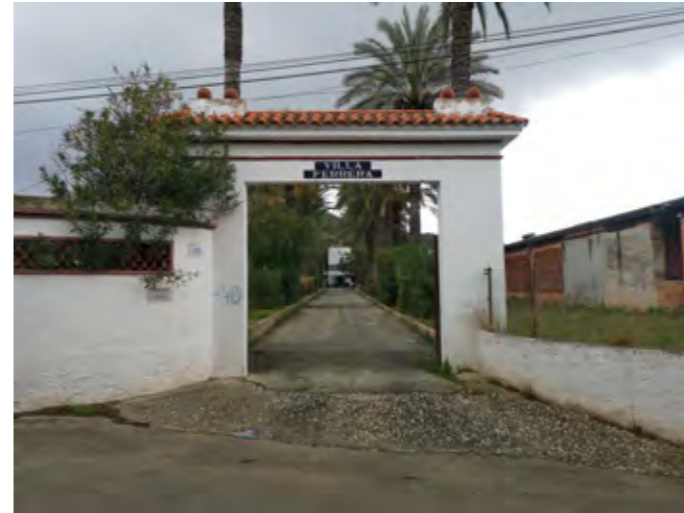
3. As I look to my left, at the end of the orange groves, there is the entrance to Villa Ferrera, a modernist gem by the architect Luis Sancho Coloma, tucked in among the factories. A somewhat curious location for a detached family house. I wonder how it was to live there when the industry was in full swing.
