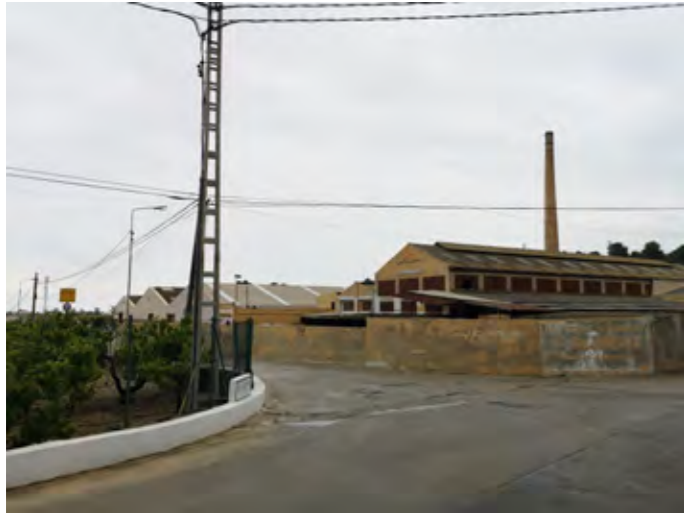
1. This walk starts at the southernmost border of Els rajolars, and goes along the area's central road, Passeig dels Rajolars. Here lays, Anticfang, the last ceramic factory in the area, still in production.
