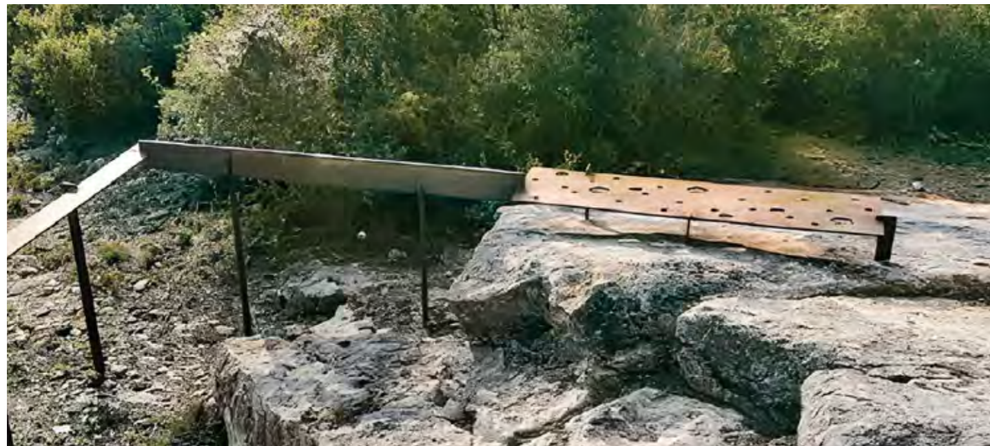
Fig. 63. Example of landscape architecture that evoke curiosity (at least with me). “Confetti” from the Girona’s Shores project by EMF. The handrail highlights the outcrop and the holes in the metal plate direct the eye towards individual fossils in the rock. Photo by: EMF
